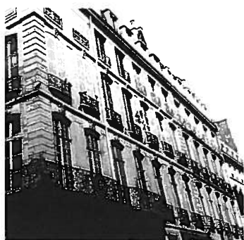
The superb wrought-iron balcony of this house situated on the corner of rue Saint-Honoré and rue des Prouvaires would certainly have overhung the shop-front of a marchand-mercier
