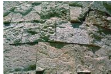
A Getty Center exterior wall faced with travertine stone. Photo: Vladimir Lange.
